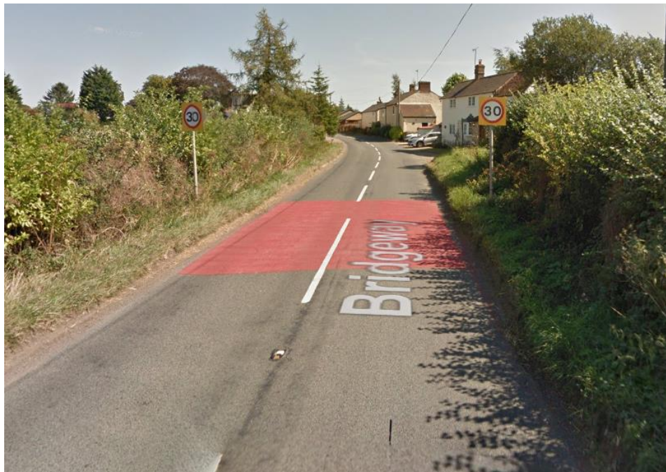
Figure 7-3 – Terminal signs on approach to the village from The Green
